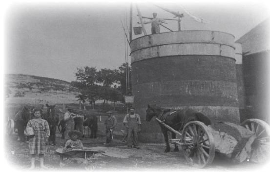
Early Poured Concrete Silo and First Ready Mixer - 1990
